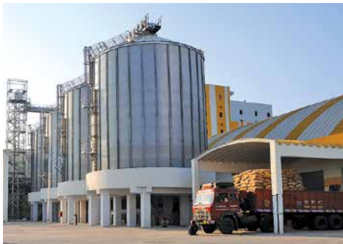
Fig. 2.8 Grain storage silo
