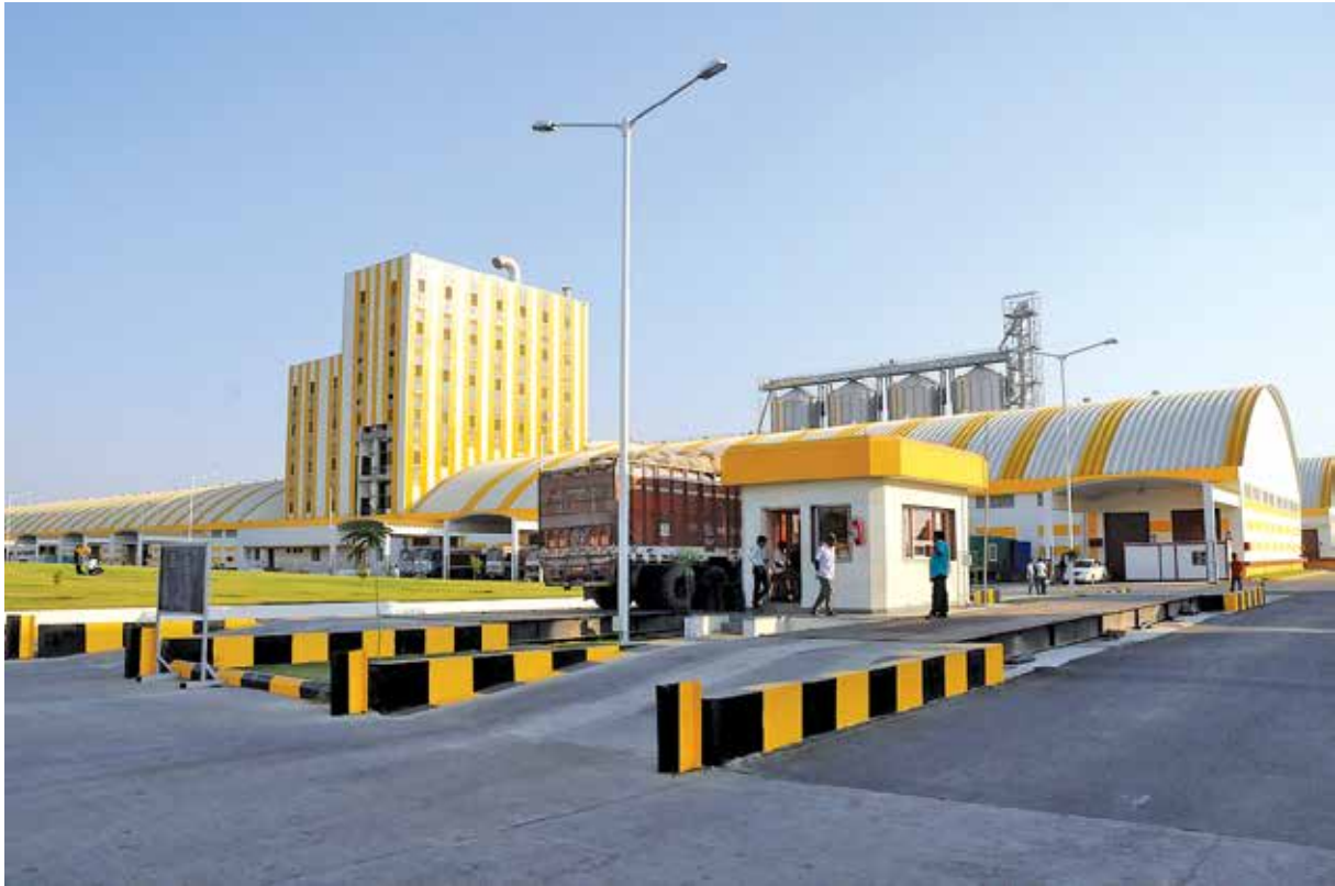
Fig. 1.0 Cattle feed plant
