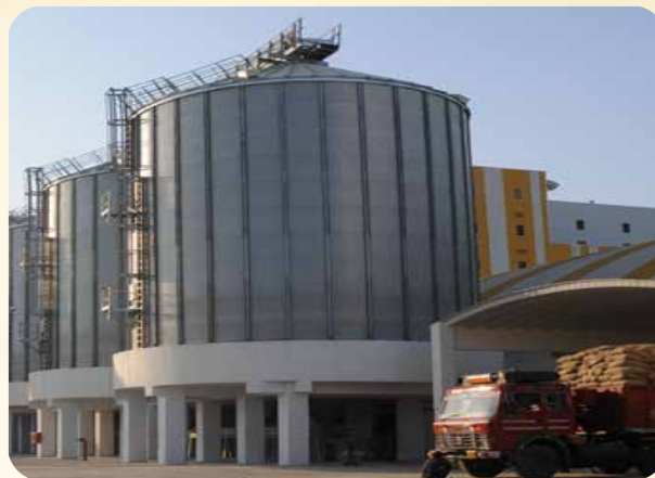
Figure 2: Grain storage silo
